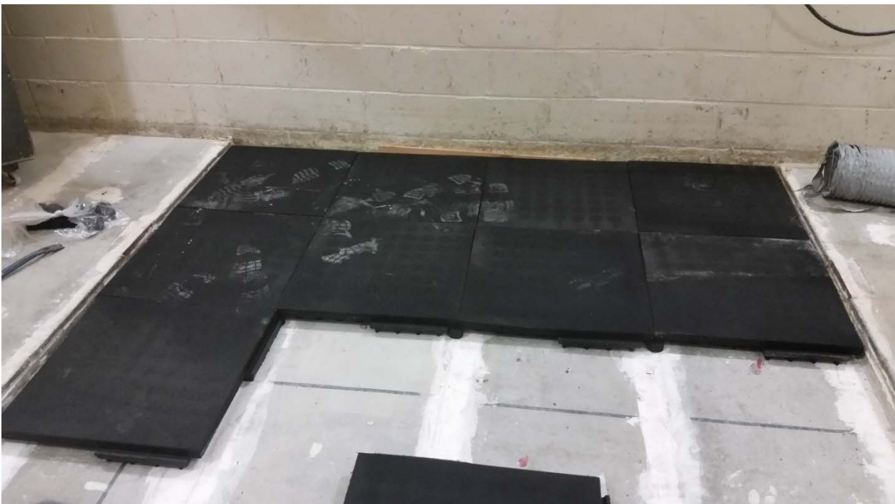
Figure 4 – Flooring partially installed
