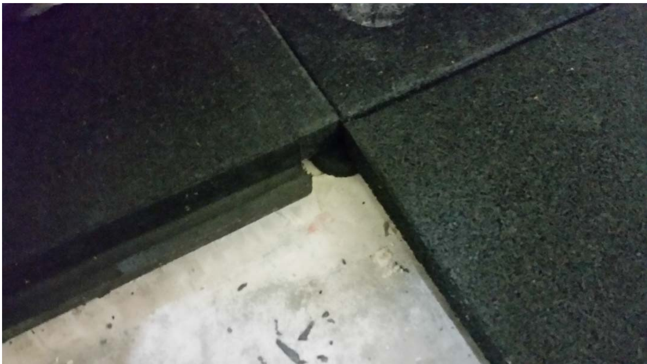
Figure 2 – Individual support pedestal installed
