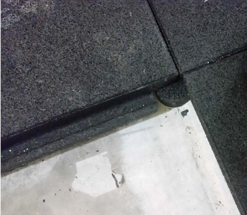
Figure 3 – Typical support pedestal installation
